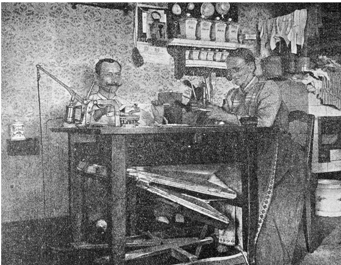
Figure 112. A hollow-beadworker's workshop (bead-molding machine with bellows) (Parkert 1925:158, Figure 37).
