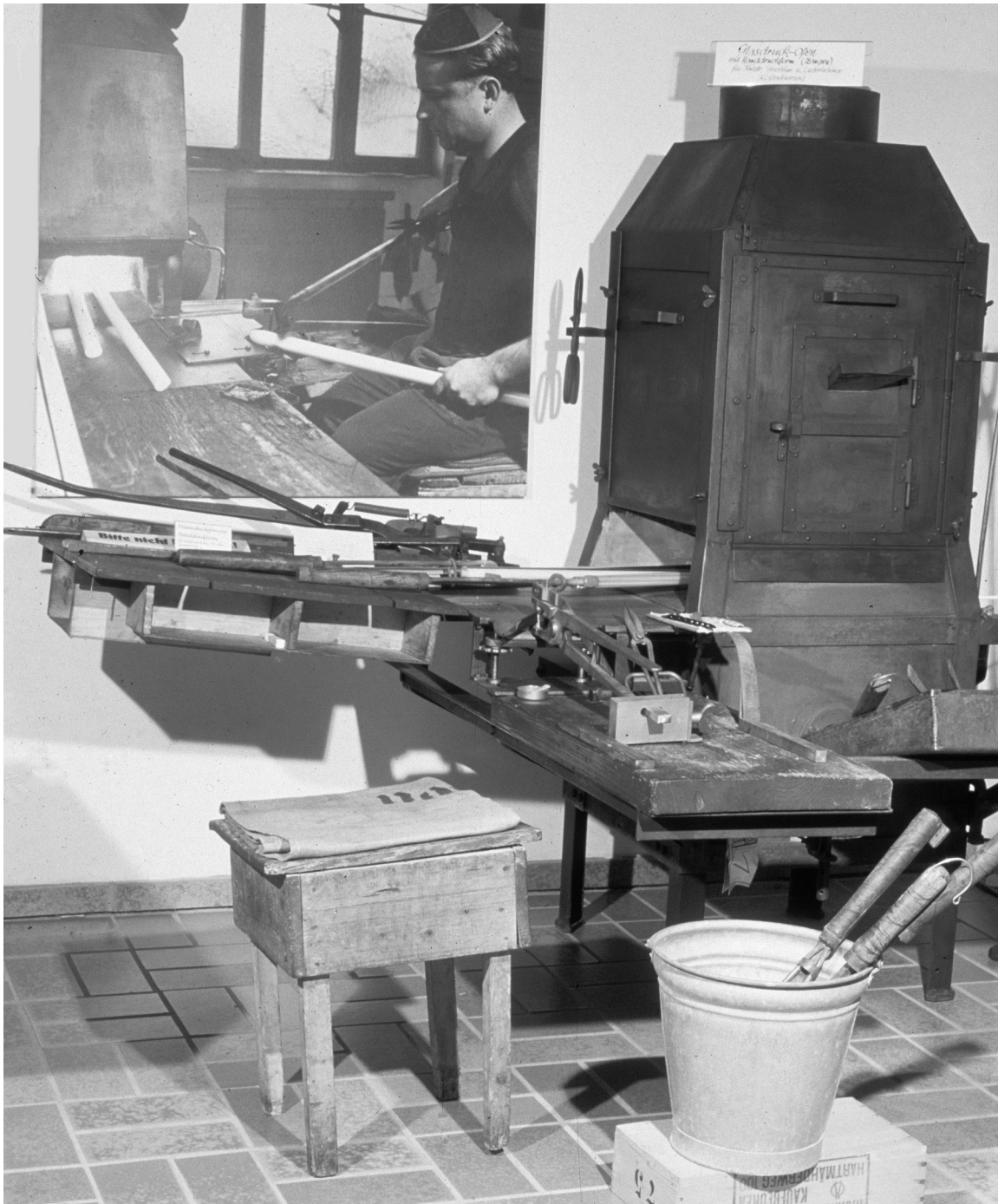
Figure 86. Press-molding work station (coal-fired furnace), Neugablonz, around 1947, with contemporary photograph (Neugablonz Industry and Jewelry Museum, Kaufbeuren-Neugablonz).
